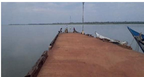
Figure 11: Harbour, where direct strainer intake was attached
