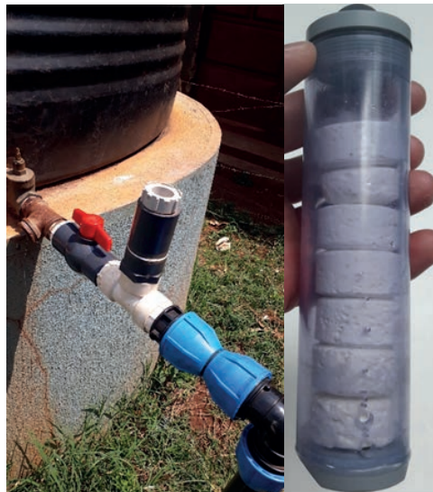
Figure 67: T-chlorinator and cylinder
